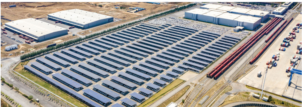
Solar panels at Tiexi plant.
